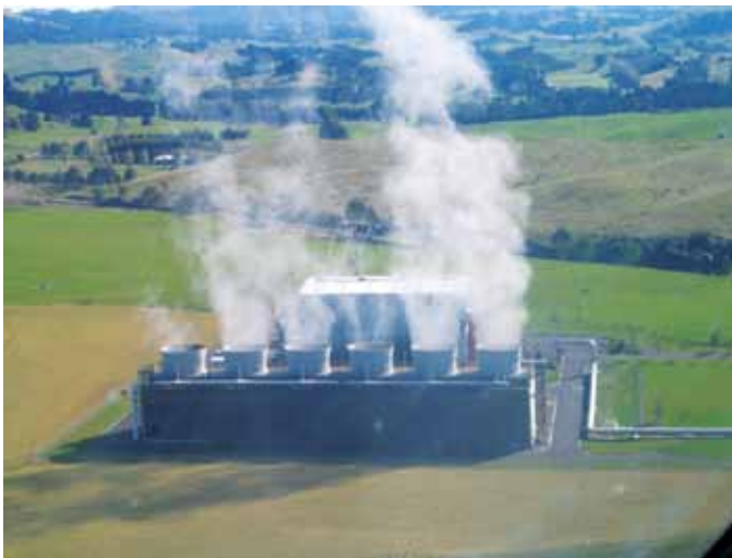
Figure A5.4: McLachlan Plant, Wairakei, New Zealand: 55-Megawatt Condensing Steam
