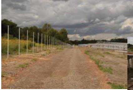
Fence and first modules
