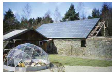
Centre for Alternative Technology Wales, UK, part of large PV-hybrid system
