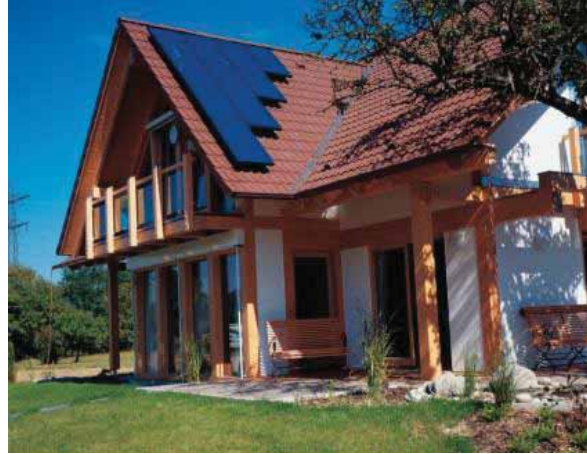
PV array on suburban house in Germany Photo: SMA Solar Technology AG
