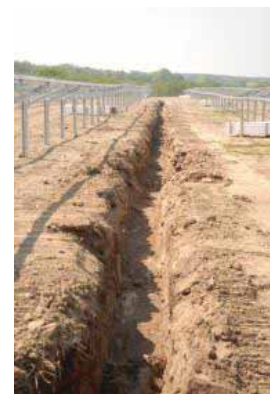
Cable laying with cable runs
