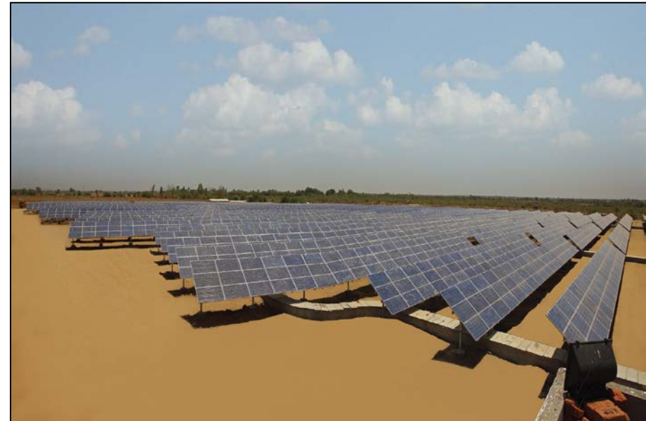
Azure Power solar panel installation in Gujarat, India
