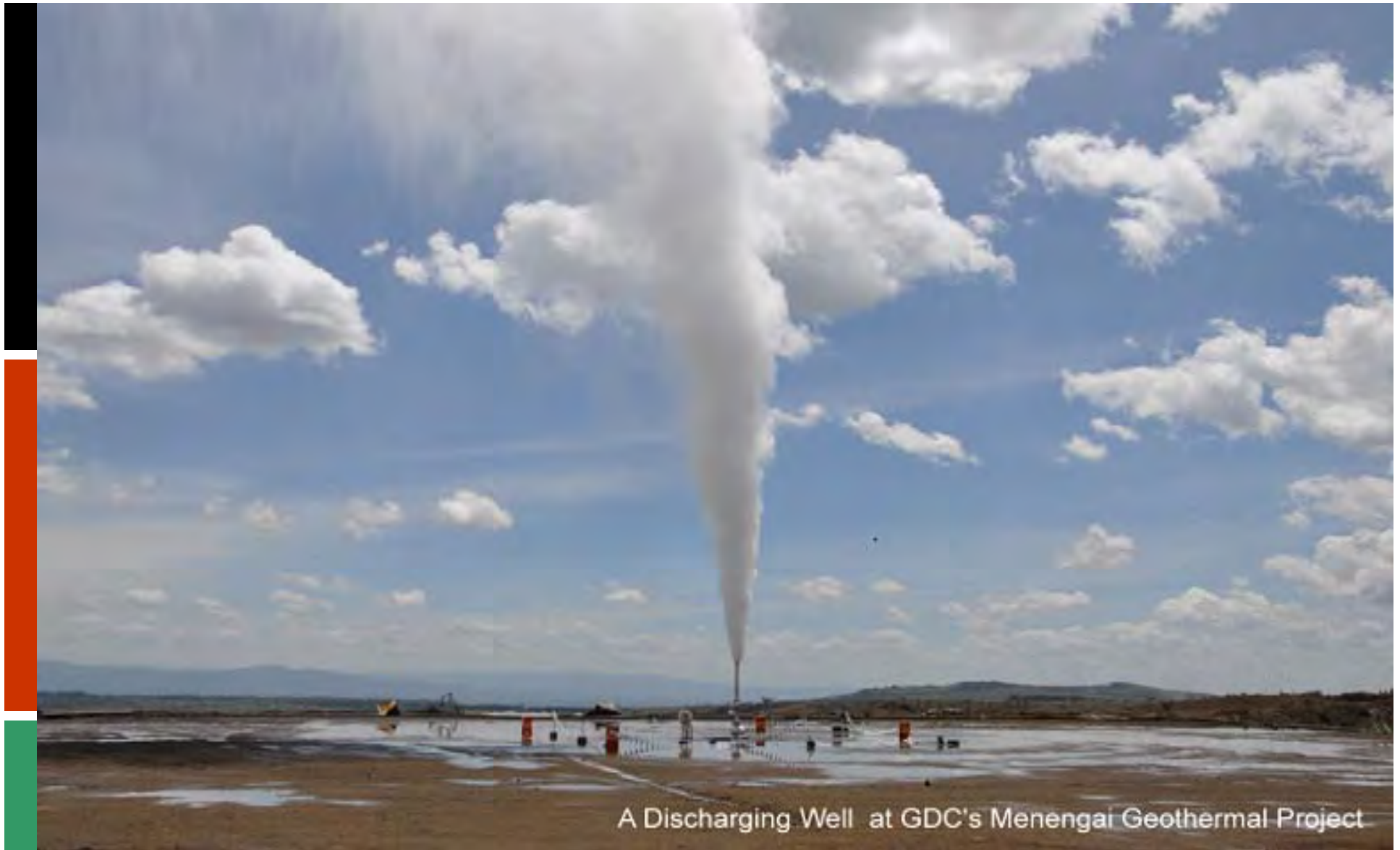
Plate 2: A discharging well at the 1600 MW Menengai geothermal field
