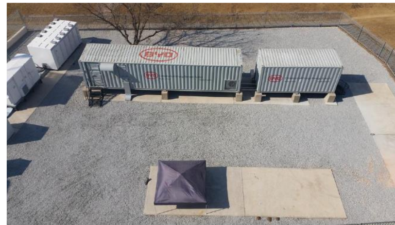
Eskom 5x200kW / 1,2MWh Experimentation Battery Site
