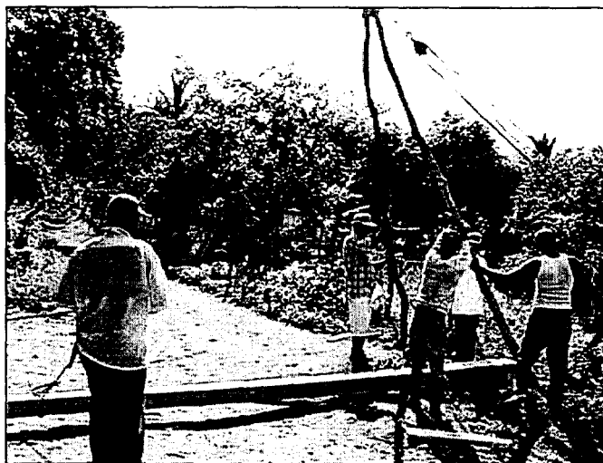
Fig. 39. A gin pole being used to raise a concrete pole. (Photo credit: Jon Katz)
