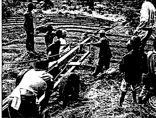
Fig. 134. Despite the use of a cart expressly built for this purpose, difficult terrain still made the task of transporting concrete poles difficult. (Photo credit: Jon Katz)
