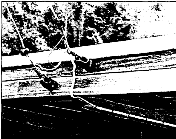
Fig. 104. The service drop fixed to the eave of the roof with wireholders.
