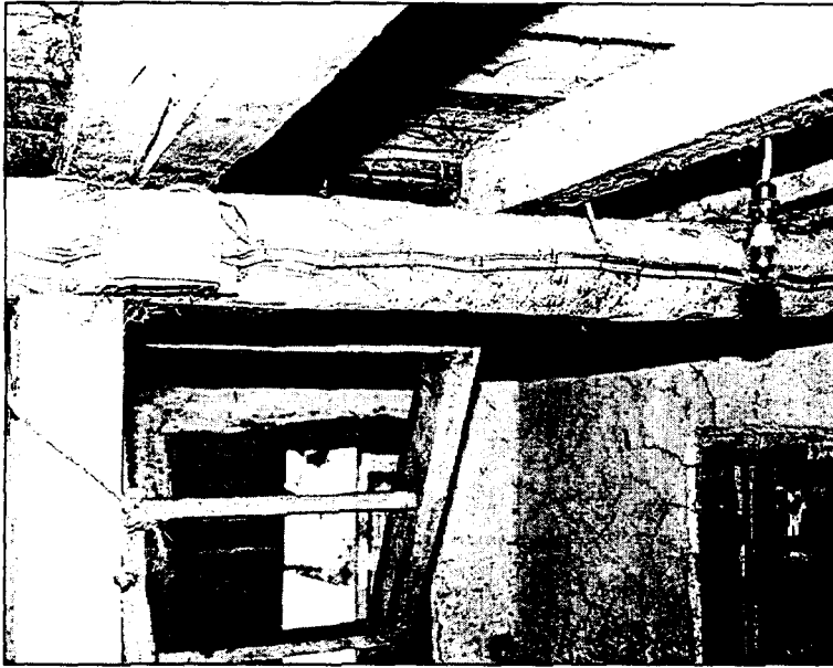
Fig. 115. Housewiring neatly stapled to beams in a home in Gotikhel, Nepal. A wooden junction box is visible in the upper left.
