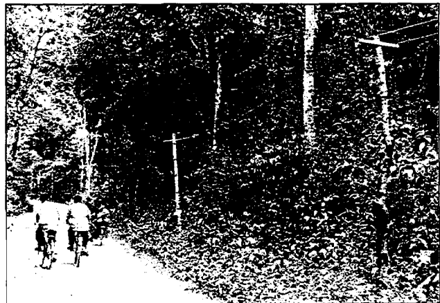
Fig. 4. The conductor used along this stretch of line between two villages is too small for the loads and distances involved.
