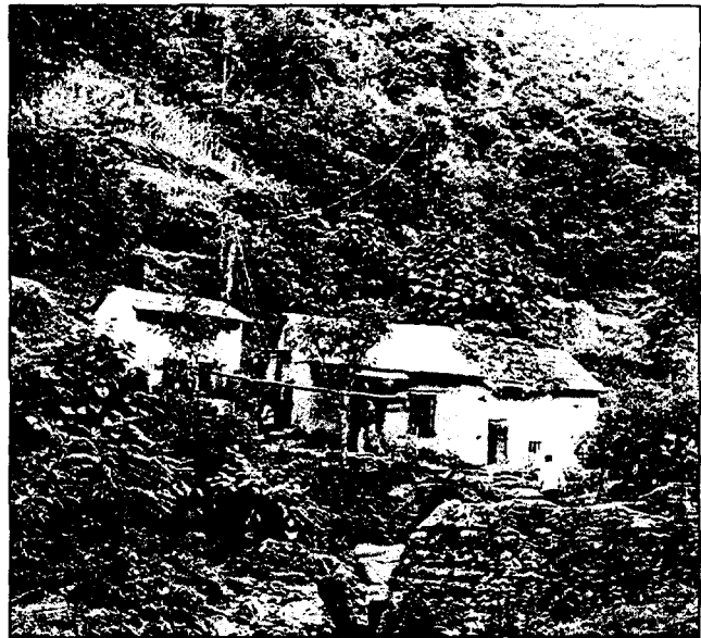
Fig. 2. A micro-hydropower plant serving remote households scattered on the hillsides near Gotikhel, Nepal.
