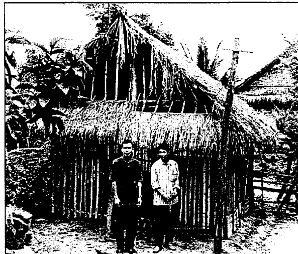
Fig. 125. Ban Nam Thung powerhouse and operators.
