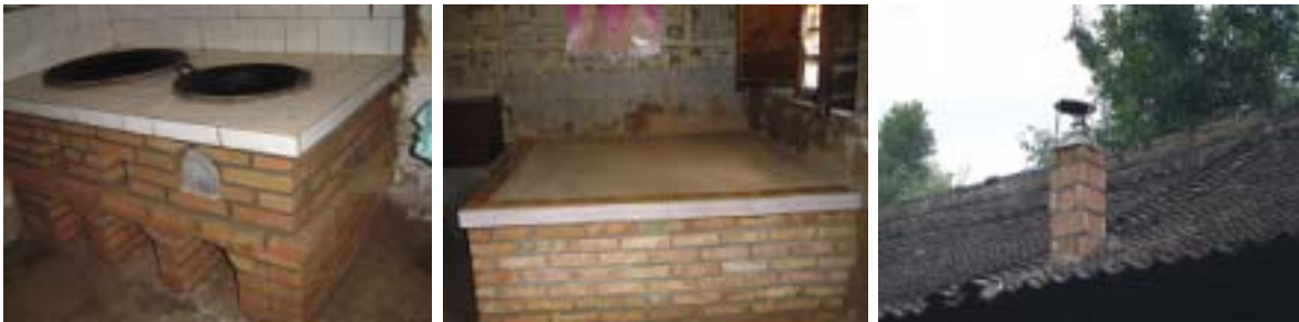
Figure 3.1b: Improved Biomass Range (left), Bed-heating Device (center) and Chimney (right), Gansu
