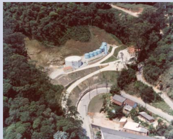
Mosela water treatment station
