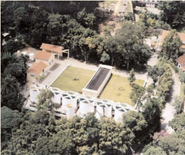
Montevideo water treatment station
