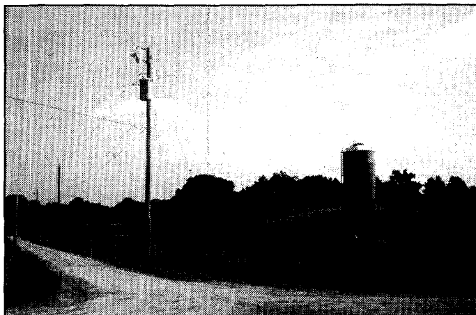
Figure 20. A 100-kVA single-phase pole-mounted transformer is adequate to serve the needs of this rural farm in the United States.
