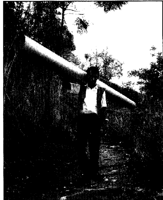
Figure 13. Sections of a steel pole fabricated in Nepal easily can be carried by porters to isolated villages.
