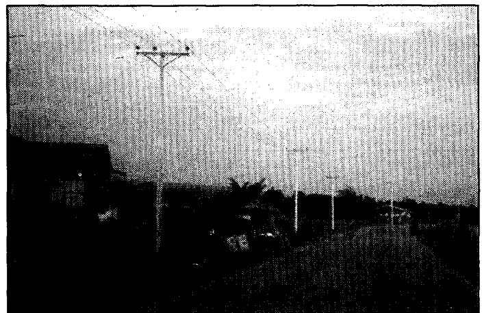
Figure 23. Even though the MV line passes by a number of households, insufficient load prevents them from receiving electricity service.
