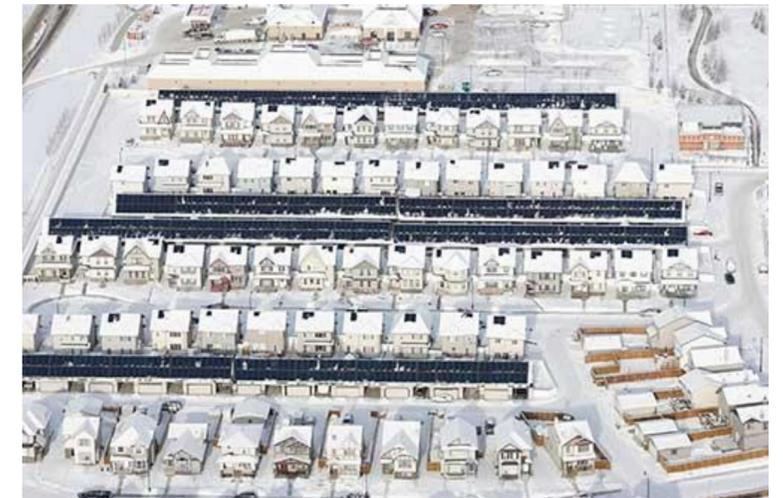
Drakes Landing Solar Community is a master planned neighbourhood that covers 90% of its energy consumption for space heating by solar energy. Seasonal energy storage is enabled by Borehole thermal energy storages. Short-term storage tanks provide a central hub for heat movement.
