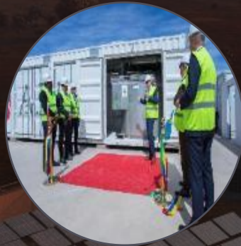
Installed and started
