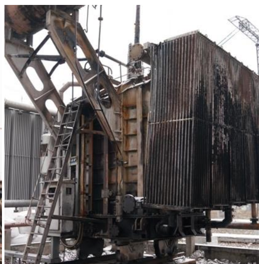
Damaged autotransformers at different Ukrenergo's substations
