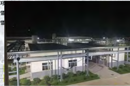
Solar P2G plant in Zhangjiakou
