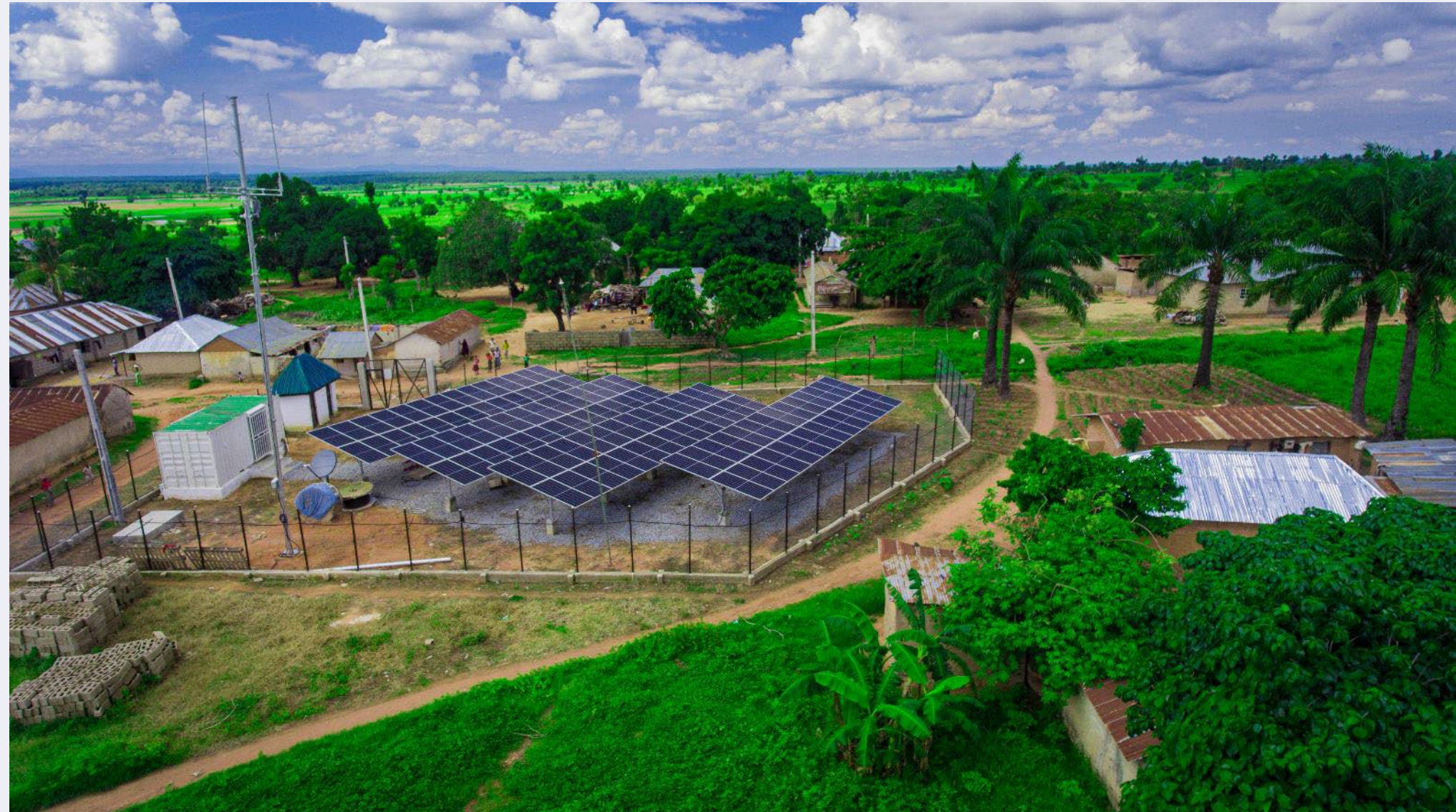
Husk's mini grid in Idadu, Nasarawa state Typical system: 30 kWp PV, biomass generator
