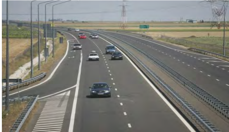
Timișoara – Arad Highway
