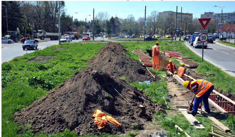
Construction site at Michelangelo passage in Timișoara
