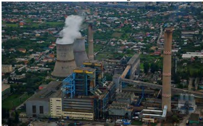
CET II District Heating Plant
