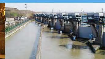
Power and Heat
