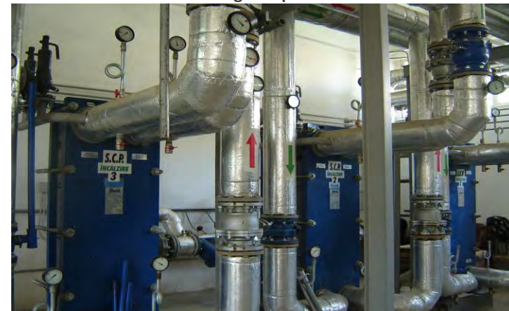
District Heating Sub-plant in Craiova
