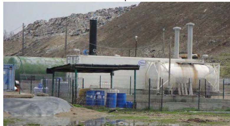
Leachate treatment plant at the landfill
