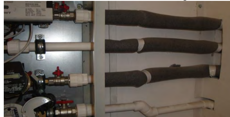
Horizontal distribution in a rehabilitated building Craiova
