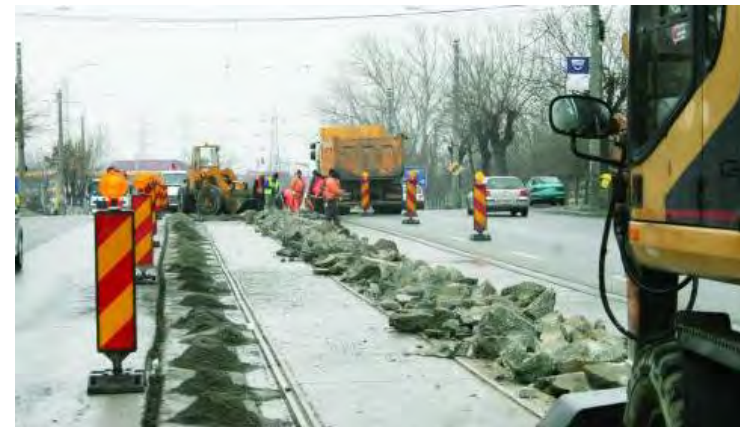
Rehabilitation of tram network in Craiova
