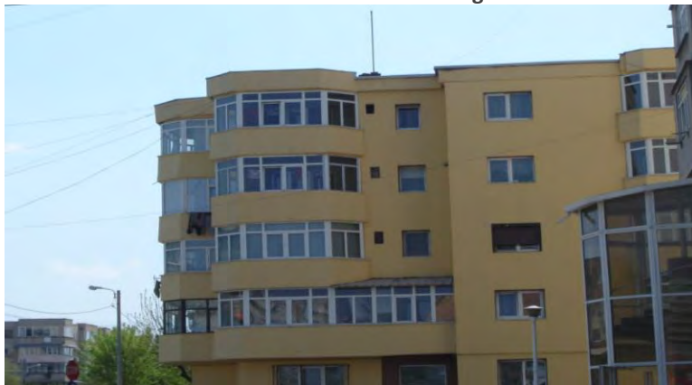
Rehabilitated residential building in Craiova
