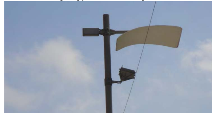
Lighting pole with switching timer
