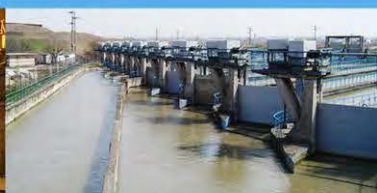
Power and Heat
