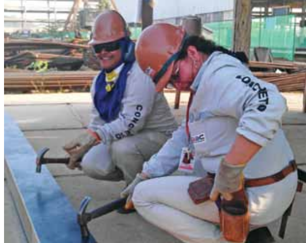
Female carpenters working on Odebrecht's Santo Antônio site, Porto Velho, Brazil. Photo: Kirsten Newitt
