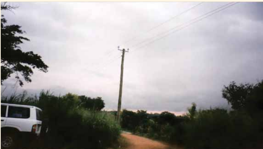
Note | A ground conductor is strung under the two insulated phase conductors, for multiple earthing. Photographed by Prof. Francesco Iliceto.
