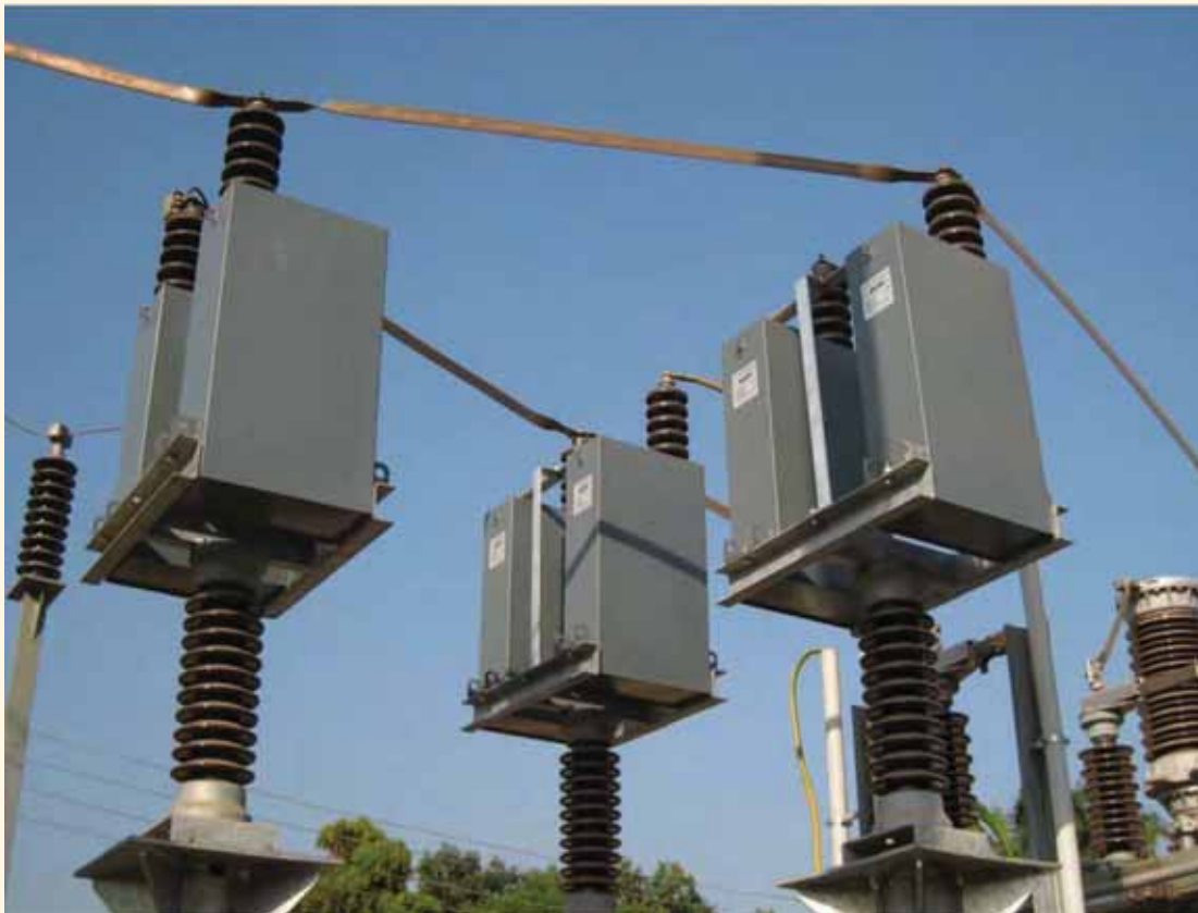
Three-Phase Capacitor Bank, Makeni, Sierra Leone
