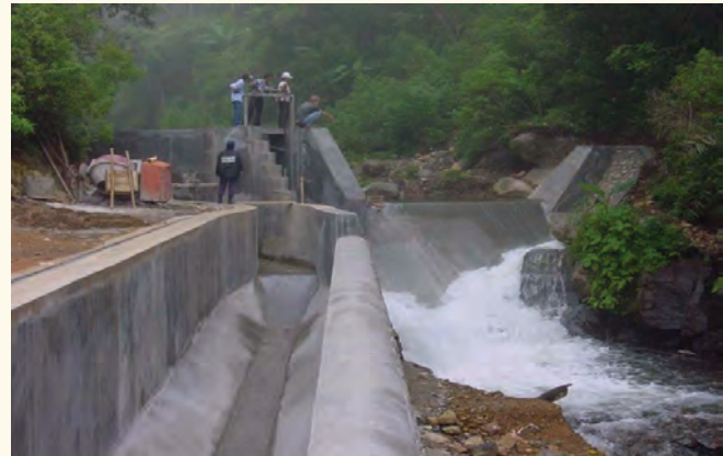
El Bote, a 930-kW hydropower project located in Nicaragua's central highlands, delivers power to 2,700 rural residents.
