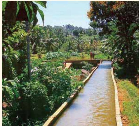
Typical village hydropower system in Sri Lanka
