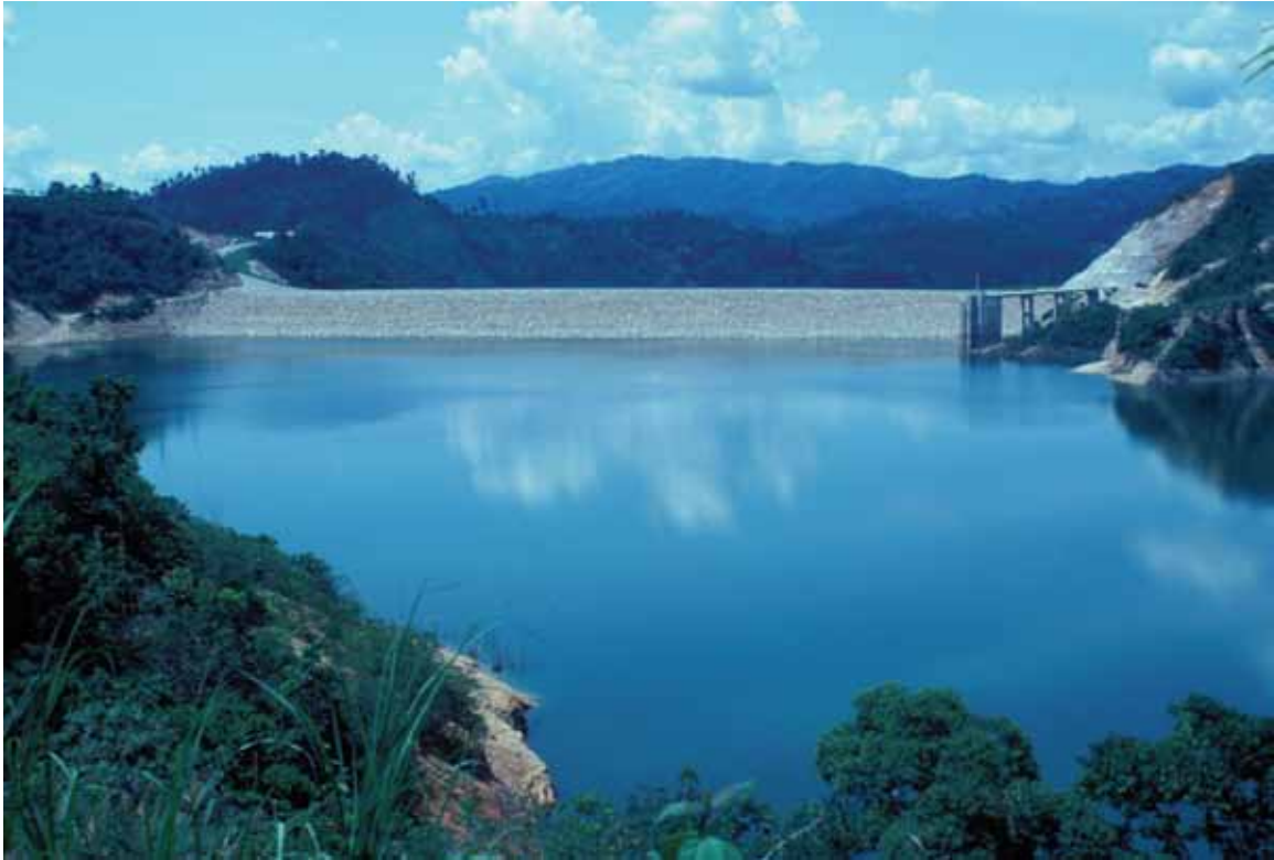
Hydropower plant in Thailand.
